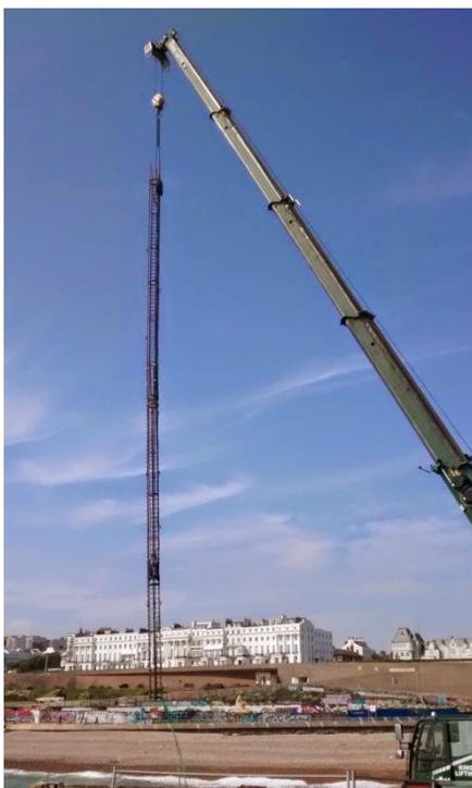
Lifting of full length reinforcing cage .
